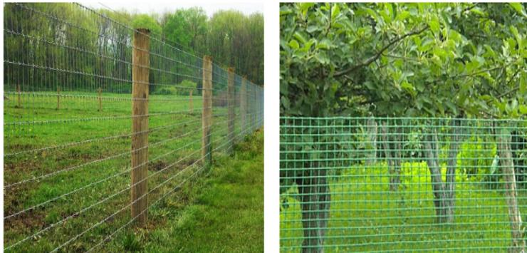
Fig. 1 Wire fence and Plastic fence
