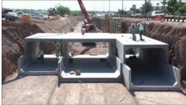
Fig. 1 precast box culvert on site (google search)
